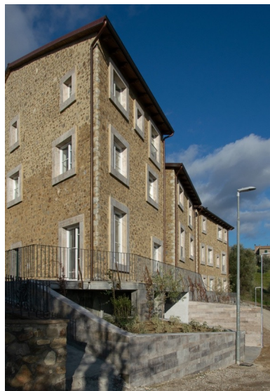
Figure 6 - 7. The project’s south front.
