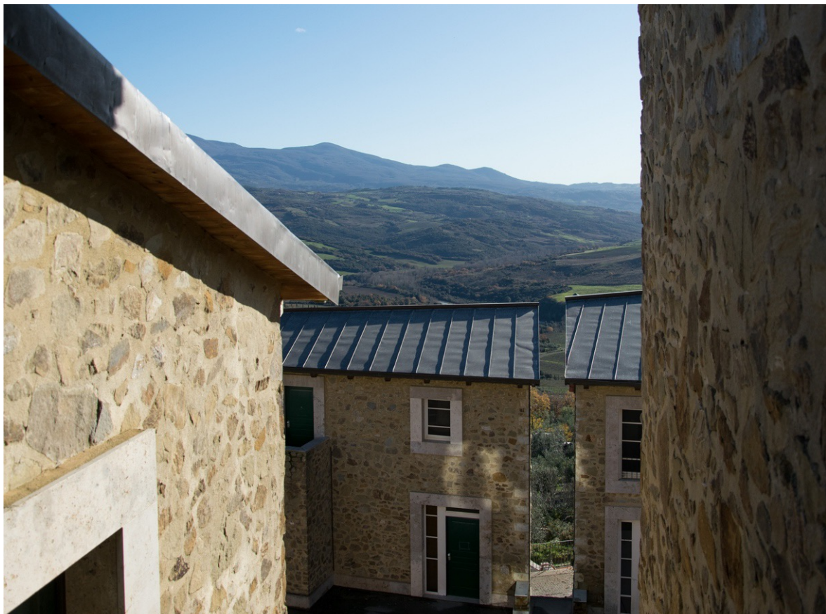
Figure 8. Views of the landscape between the blocks.
