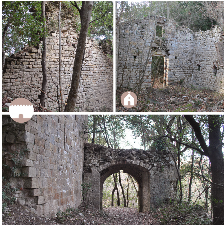
Fig 5. Views of the boundary wall and the church.
