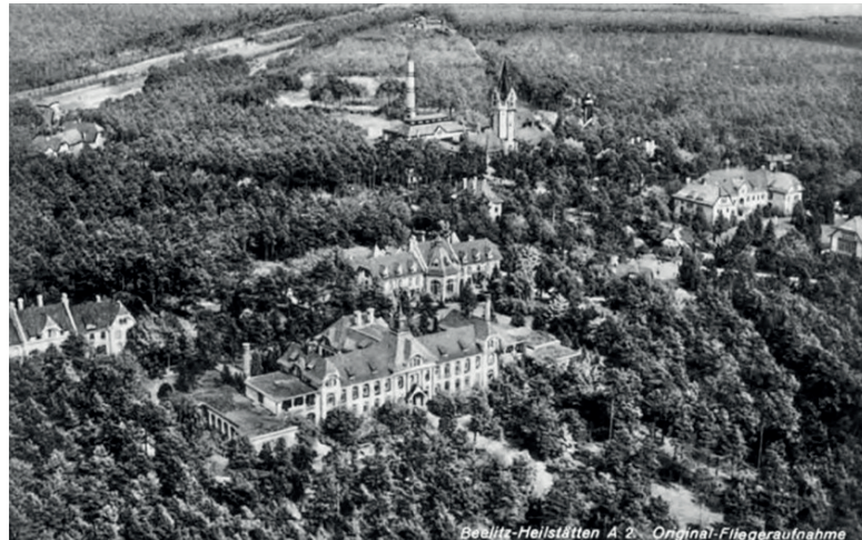
Figure 4. Site plan of the Beelitz sanatoriums, 1927, and Historical photos of the buildings into the extensive park forest. In the foreground the women's sanatorium, 1935.
